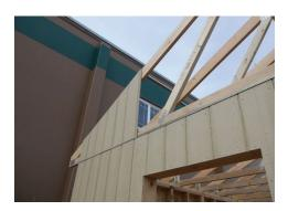
**Note:** the sheets don't go all the way to the end of the truss. These are filled in later with small pieces. Start even with the edge of the wall. Mark your cuts for the gable end vent on the outside under the peak where you want it to go. Cut siding out and caulk vent in place.
