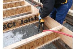
center them on the marks. Attach with 4-10d common galv nails on each top and 2 on the face on the rim boards.
