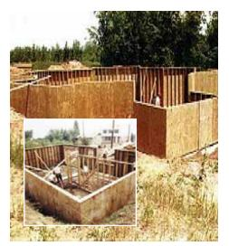
**Permanent Wood Foundation (PWF) System** is a treated plywood and lumber foundation that installs in any weather. Builders have discovered advantages to include: savings in scheduling; installation by carpentry crews; reduction in material costs, especially where concrete is at a premium, and easy to insulate and finish as a conventional frame wall. The PWF system is all about quality, strength, ease of installation and comfort.
